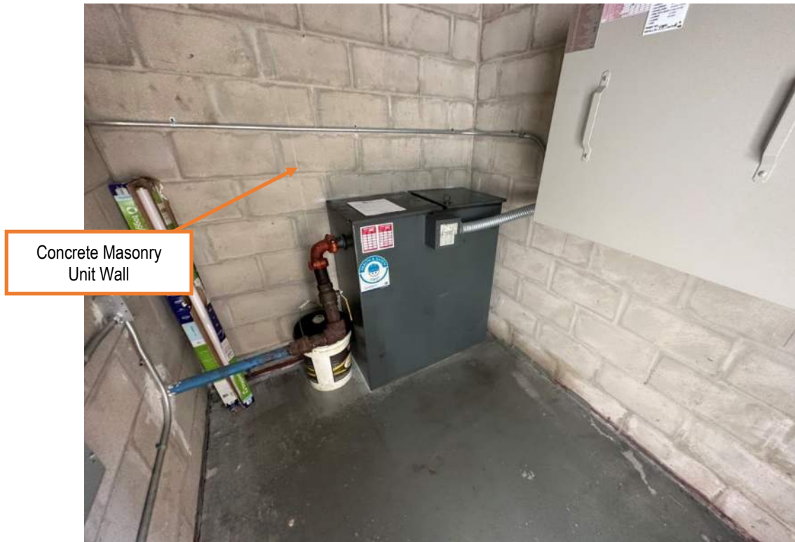
Figure 5: Elevator Machine Room
